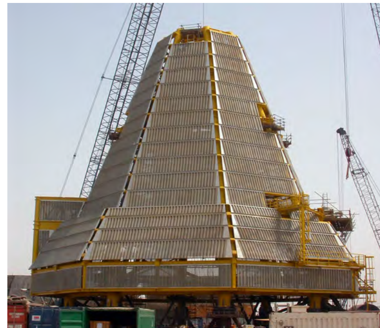
Right top picture: SBM – White Rose – Turret Heatshields
