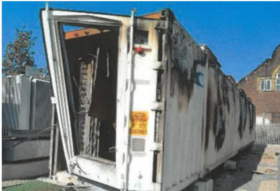
**BESS Thermal Runaway Event (No Blast / Explosion Relief Installed)**
