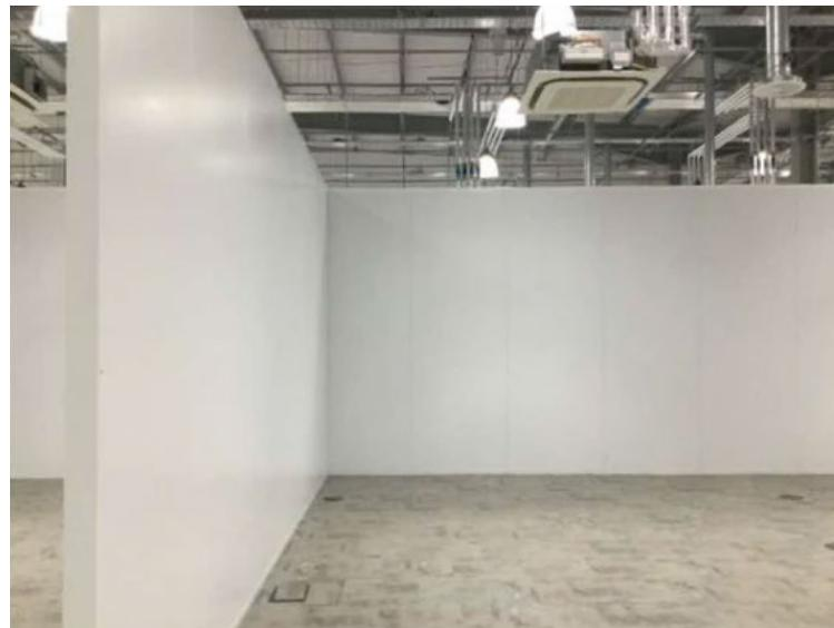
The panel thickness can be increased to provide for additional thermal or acoustic requirements, without having to add cumbersome and expensive secondary layers of panels. The standard system is made up of 550 mm wide panels which can span 3m in height without the need for secondary support steelwork.
